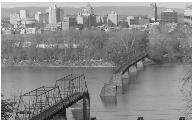
HAER documentation photo of Walnut Street Bridge, Dauphin County
