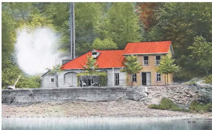
Historic Postcard of a pump station in Clarion County
