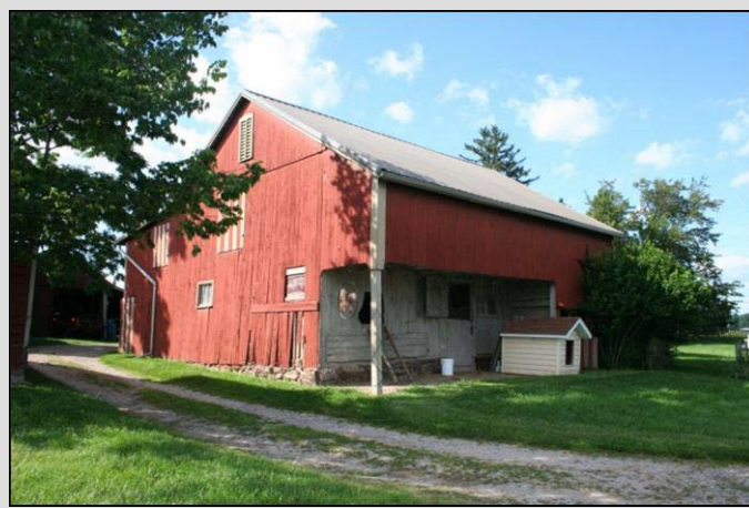
Ground barn with partial forebay, Reading Township, Adams County, c. 1880-1900. Site 001-RE-006.
