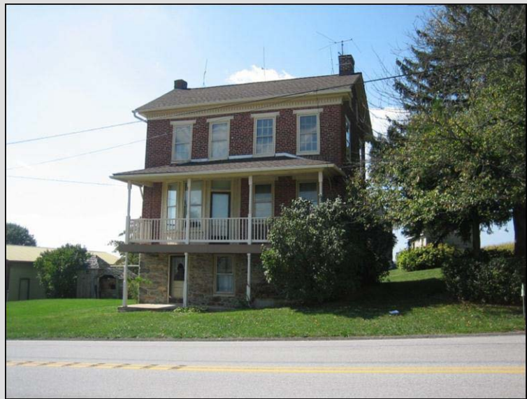
Four bay, three level house with walk in lower level and double decked porch, Codorus Township, York County, c. 1850. Site 133-CO-003.
