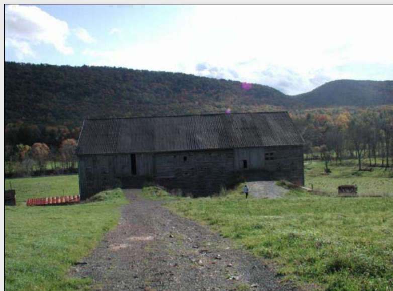
Hodge Barn, Centre County, struts under forebay
