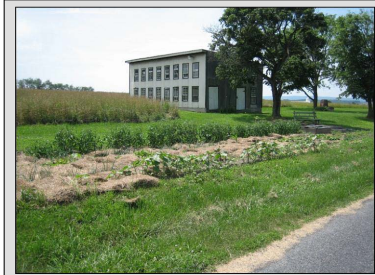
Poultry housing, Straban Township, Adams County, c. 1940-60. Site 001-ST-003.
