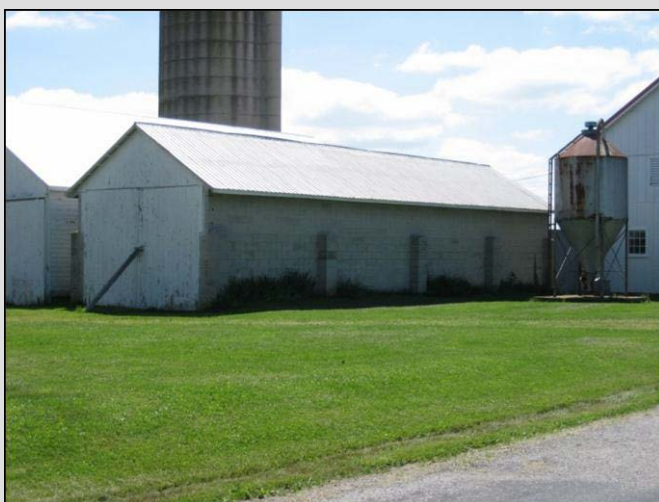
Horizontal silo, Latimore Township, Adams County, c. 1955. Site 001-LA-012.
