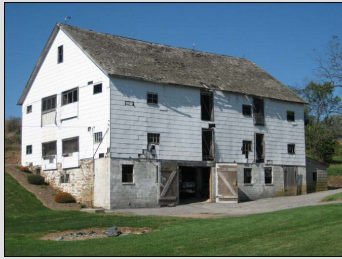
Pennsylvania forebay barn adapted for poultry housing, Codorus Township, York County, original construction c. 1860, altered for poultry in the twentieth century. Site 133-CO-008.
