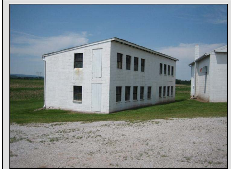
Poultry housing, Straban Township, Adams County, c. 1945-60. Site 001-ST-002.
