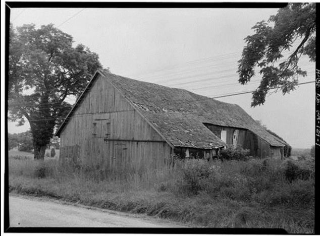
Ground barn, Dover, York County, date unknown, but possibly c. 1830. Historic American Buildings Survey. Reproduction Number: HABS PA,67-DOV,1--1
