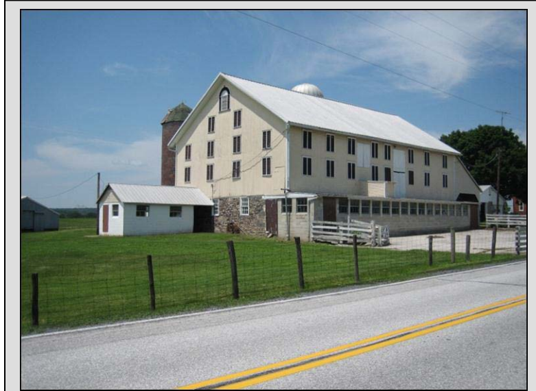
Pennsylvania forebay bank barn with forebay side extended and enclosed to accommodate more dairy cattle, Straban Township, Adams County, built 1875, altered c. 1950. Site 001-ST-002.
