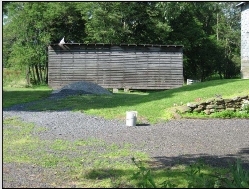
Shed roof wood slatted corn crib, Mount Joy Township, Adams County. Site 001-MJ-003.
