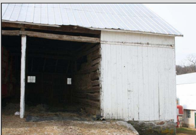
Log crib in a Pennsylvania forebay barn, Codorus Township, York County, c. 1820-40. Pierceville Run Historic Agricultural District.
