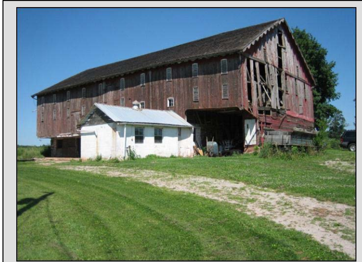
Pennsylvania forebay bank barn with integral machinery bay, Tyrone Township, Adams County, c. 1880. Site 001-TY-003.
