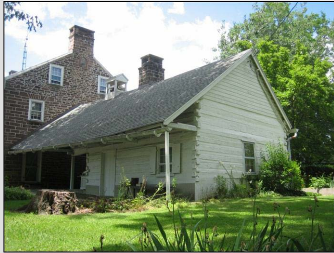
Log kitchen, Latimore Township, Adams County, early 19 th century. A large beehive oven protrudes from the end nearest the house. Site 001-LA-005.
