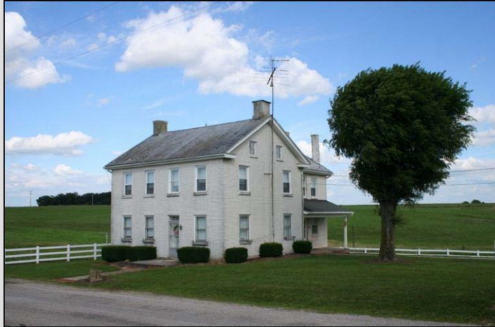
Four-over four, double pile Pennsylvania Farmhouse with single off-center door, Reading Township, Adams County, c. 1850. Site 001-RE-005.
