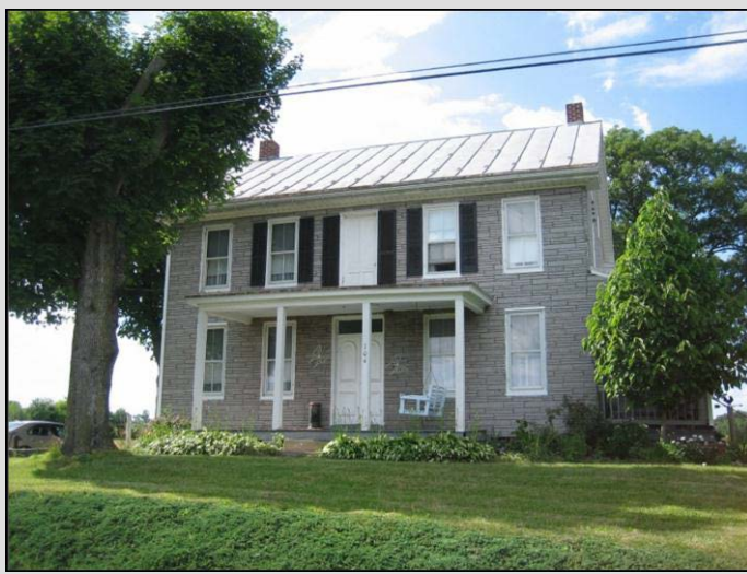
Five-bay, center door house with Italianate trim, Mount Joy Township, Adams County, c. 1870. Site 001-MJ-003.
