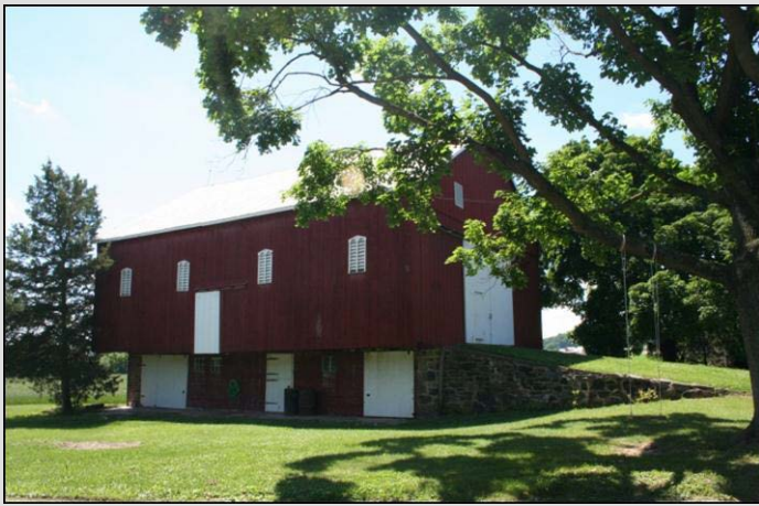
Pennsylvania forebay barn with ramp in the gable end, Reading Township, Adams County, c. 1875-1890. Site 001-RE-004.
