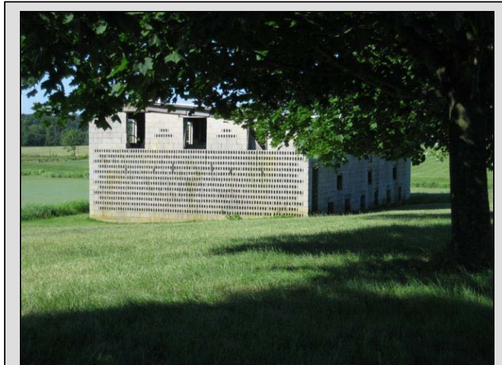
Poultry house with hollow concrete block corncrib at one end, Tyrone Township, Adams County, c. 1960. Site 001-TY-001.
