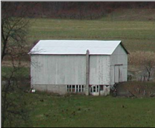
Lancaster County style tobacco barn near Kantz, Snyder County, c. 1940. Photo taken from road by Sally McMurry; no site number.
