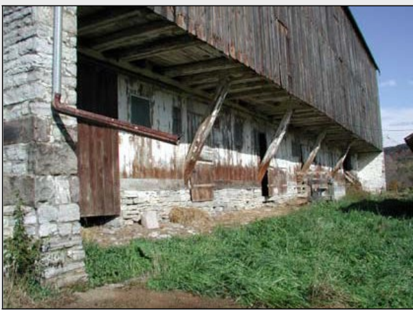
Hodge Barn, Centre County, struts under forebay
