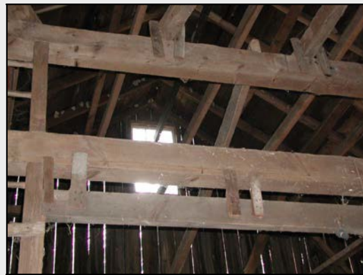
Interior of a Pennsylvania barn showing the cleats on the upper beams which hold tobacco laths in place, West Lampeter Township, Lancaster County, c. 1875.
