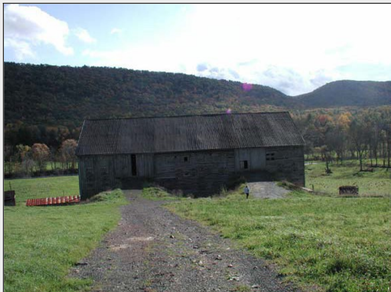
Hodge Barn, Centre County, struts under forebay
