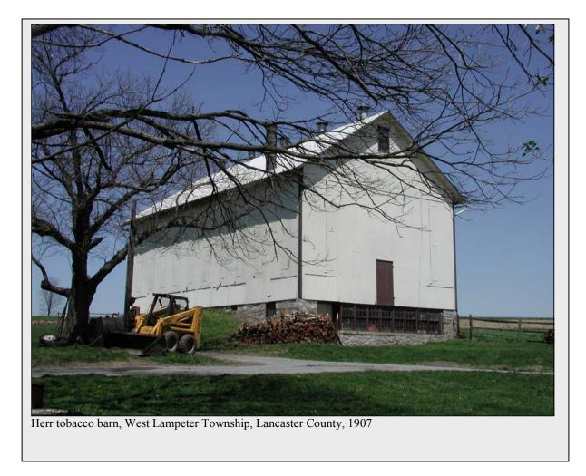
This barn has vertical slats, metal ventilators, and a gable-end stripping room. The vents are closed in this photo.
