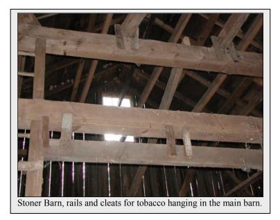
Though separate tobacco barns were common, some farmers adapted their main barns. They might add onto one end of a larger barn, or mount "cleats" on threshing floor level framing members to receive tobacco rails.<sup>89</sup>
