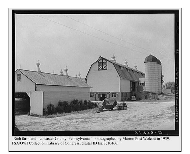
This is a good example of a barn that conformed to new ideals in barn design. The lower level is built of concrete block. It is liberally pierced with large windows and organized lengthwise. The upper level has a gambrel roof for extra hay storage.
