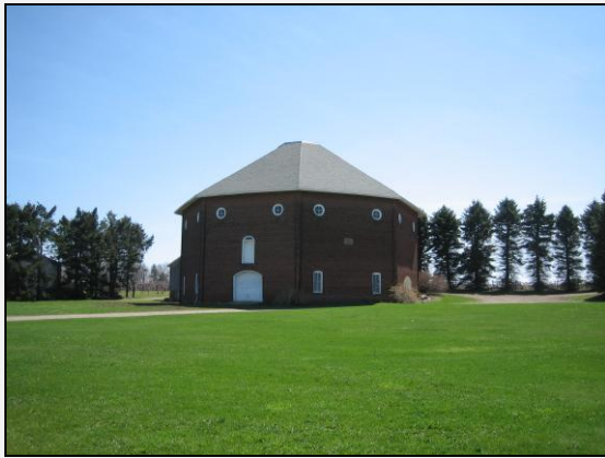
Octagon Barn, North East Township, Erie County, 1879. Site 049-NE-002.
