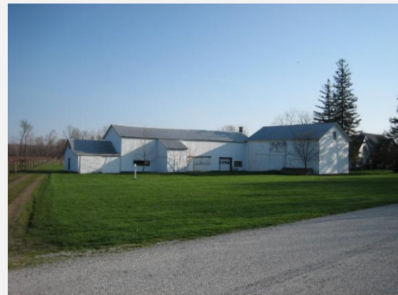
English barn with packing house extension, North East Township, Erie County, original 19th century, addition early 20th century. Site 049-NE-006.
