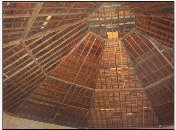
Octagon Barn Interior, North East Township, Erie County, 1879. Site 049-NE-002.
