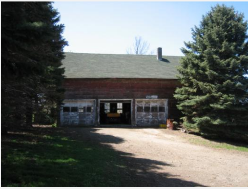
Packing house converted to migrant quarters, North East Township, Erie County, original construction c. 1920, conversion c. 1955-60. Site 049-NE-002.
