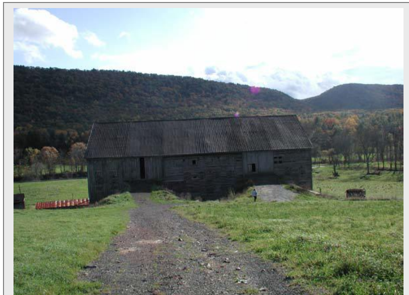
Hodge Barn, Centre County, struts under forebay
