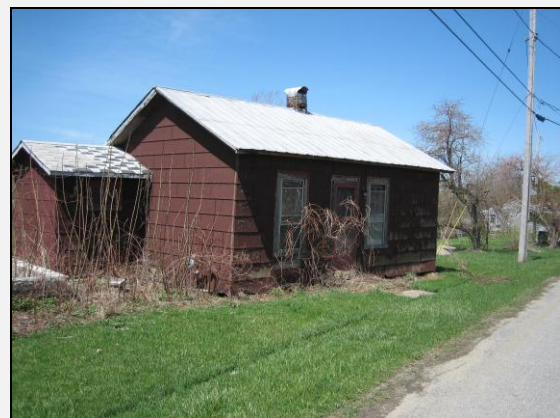
Probable tenant house, North East Township, Erie County, c. 1920-40. Site 049-NE-001.
