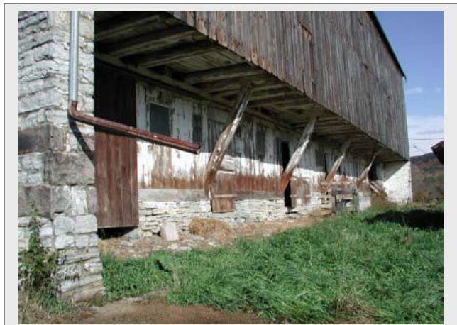
Hodge Barn, Centre County, struts under forebay
