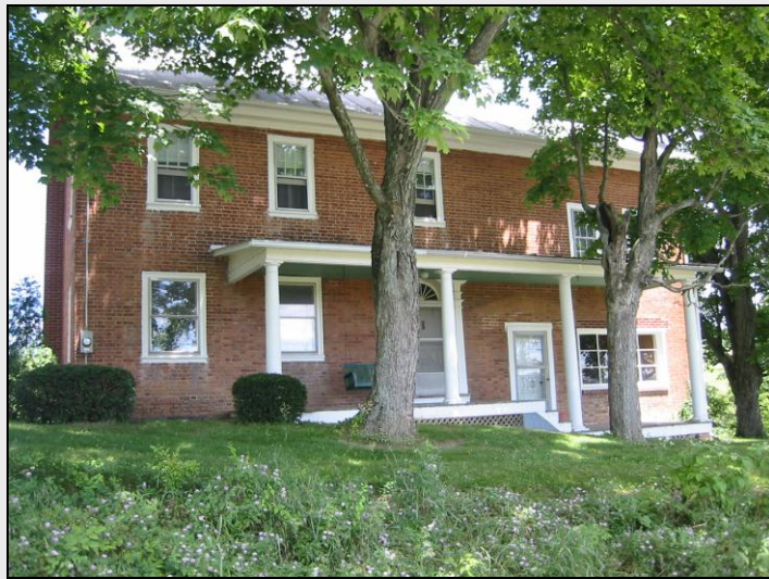
Brick three-bay house, Greenwood Township, Columbia County, c. 1830. Site 037-GR-003.
