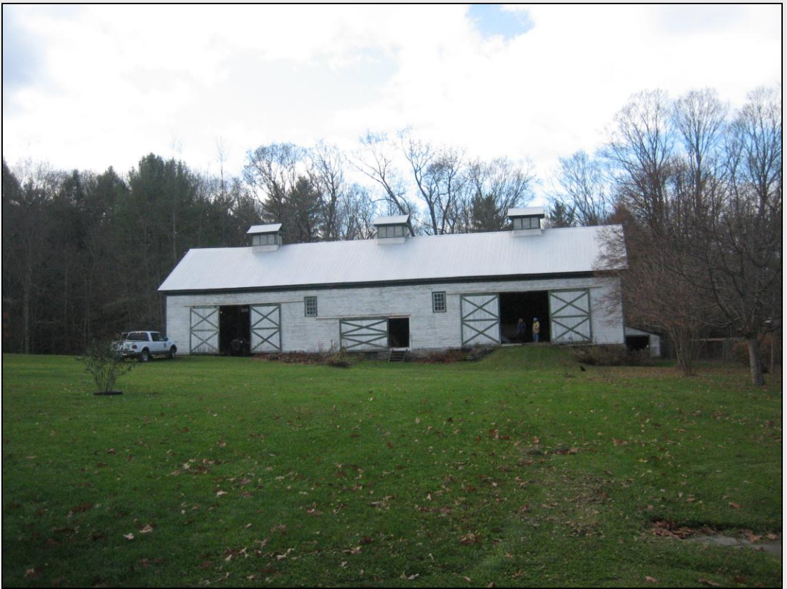
Barn near Towanda, Bradford County. Two early English barns were connected and ventilators added later. Photo-only site, no site number.
