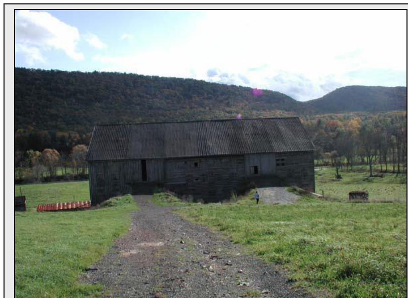
Hodge Barn, Centre County, struts under forebay
