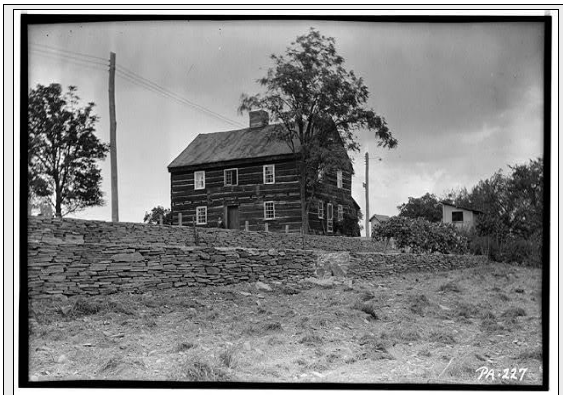
Center chimney New England-style log house, Terrytown, Bradford County, c. 1806. HABS, photographed by Stanley Jones in 1936.
