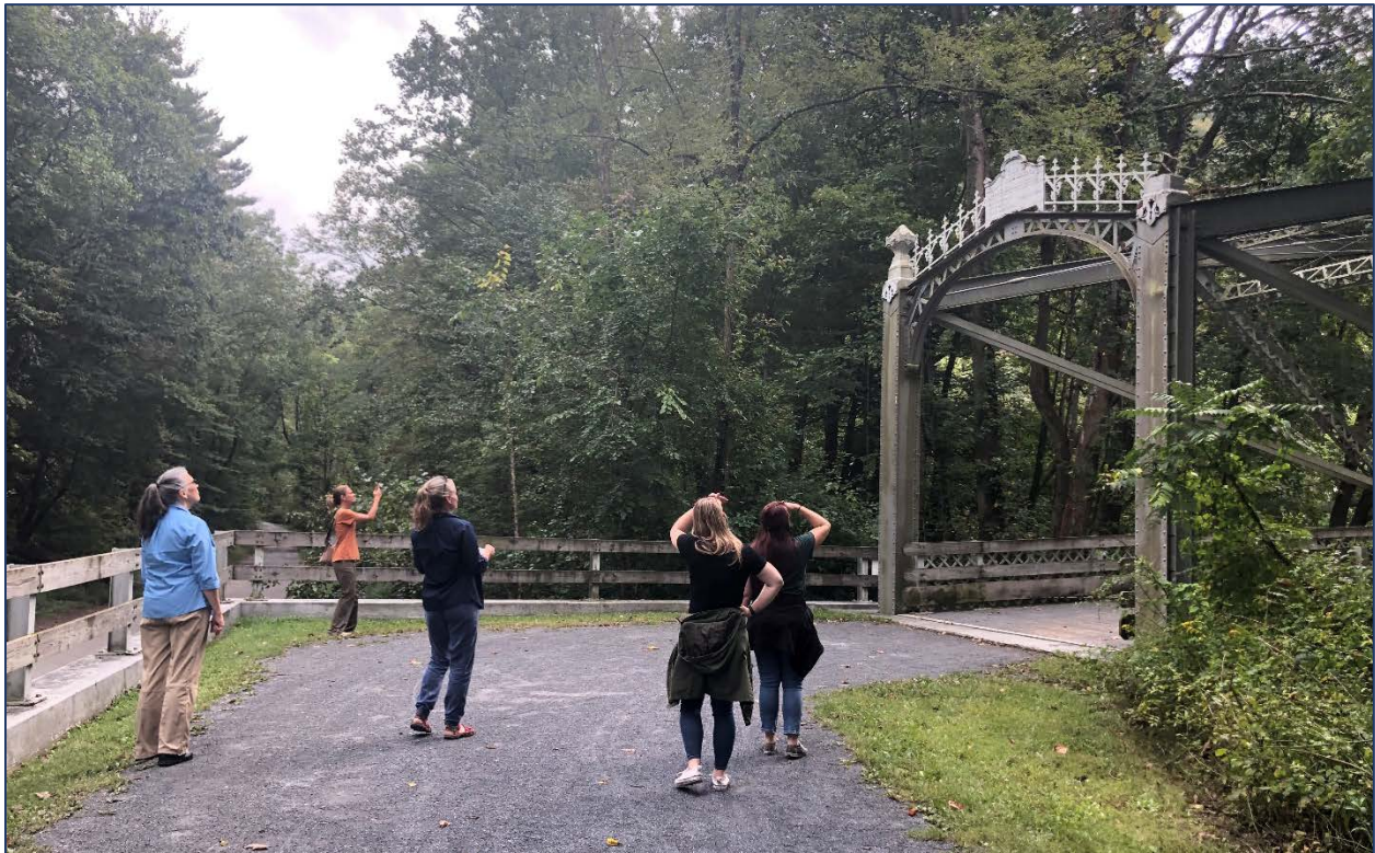
Figure 9: A group of PA SHPO staff enjoying a historic metal truss bridge in Lebanon County, P.A.
