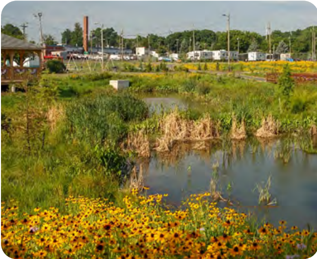
Example of Green Infrastructure Site, Park and Drainage Integration. A larger water retention program can assist with riverine flooding. These constructed natural areas support pollinators and local animal life, while also reducing flooding upland.
