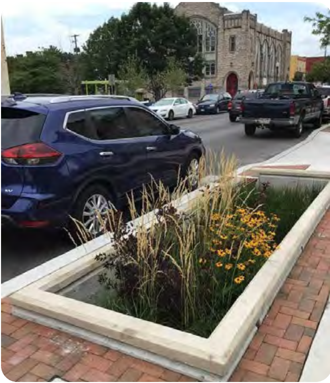
Examples of Green Streets, Improved Drainage, Storm water Storage and Street Landscaping. Green storm water infrastructure effectively reduces flooding while also improving the public realm. Green space and sidewalk bump outs beautify the sidewalk and slow traffic.
