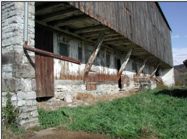
Hodge Barn, Centre County, struts under forebay
