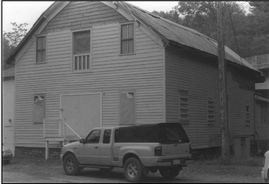
Exterior of the Metz ice plant, Pike County, c. 1869. Pennsylvania Historic Preservation Bureau file photo.
