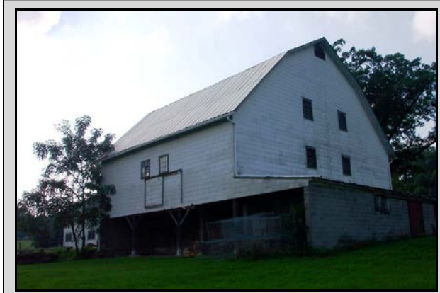
Pennsylvania forebay barn with gambrel roof, Dallas Township, Luzerne County, c. 1900. Site 079-DA-002. It is not known if the gambrel roof was original, or a later alteration.
