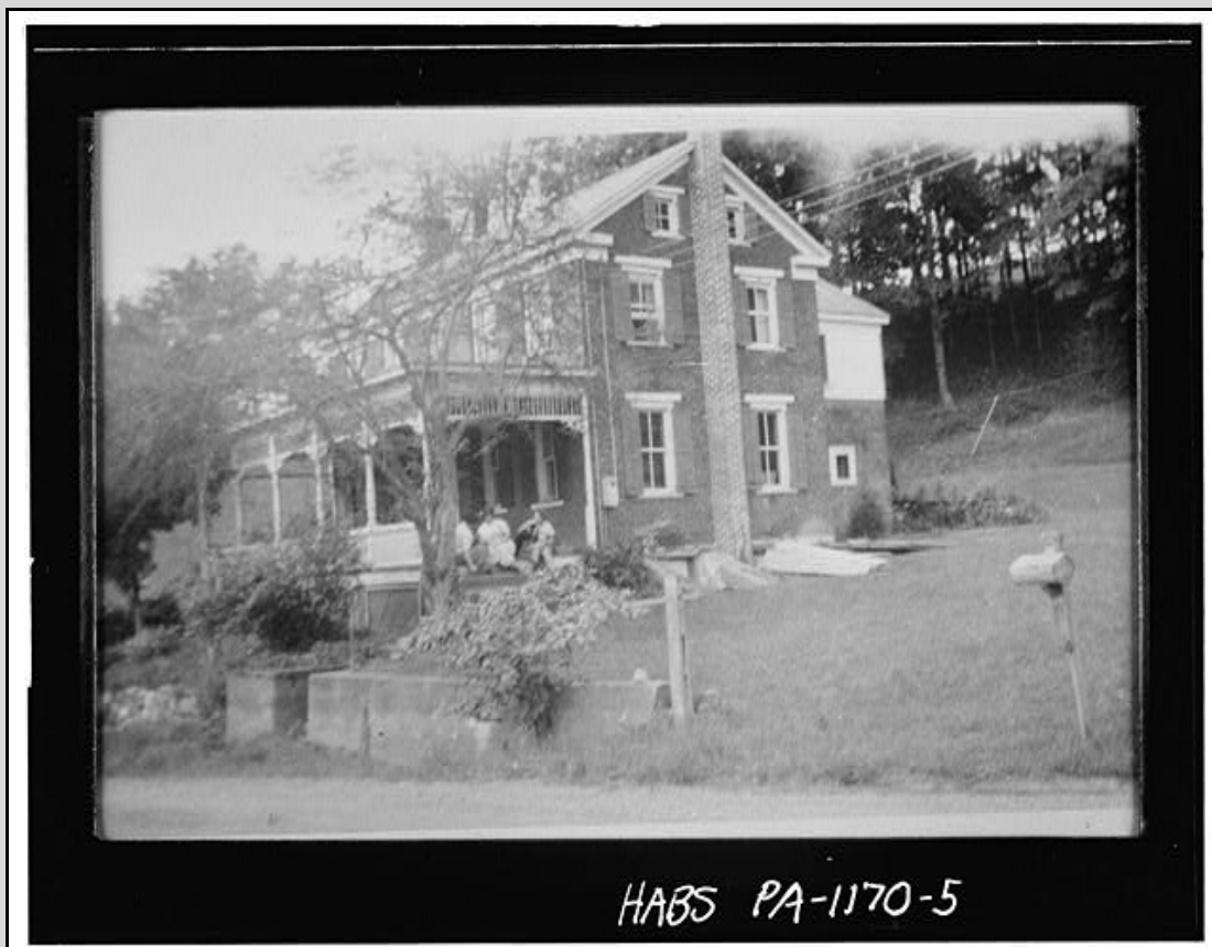
Samuel Michael House, Middle Smithfield Township, Monroe County, built mid- century; a porch added in the 1890s; this was replaced in the 1930s by the owner, Chauncey Dimmick, and at about the same time the rear ell was raised to two stories and an external stair access to the second floor added. Photocopy of photograph from the collection of Mr and Mrs John A. Farrington, Lititz, Pa. Photographer: unknown; date, about 1935. Recorded by the Historic American Buildings Survey. Digital ID http://hdl.loc.gov/loc.pnp/hhh.pa0601 . The owner from 1900 to 1937, Chauncey Dimmick, was a farmer with 136 acres. His year-round household had only two people, so it is very possible that the alterations were made for summer boarders.
