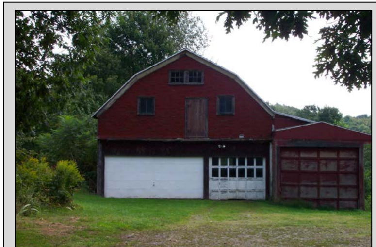
Possible fruit packing house, converted to garage, c. 1930-50, Newton Township, Lackawanna County. Site 069-NE-001.
