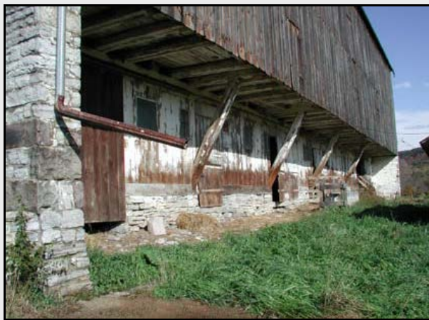
Hodge Barn, Centre County, struts under forebay.
