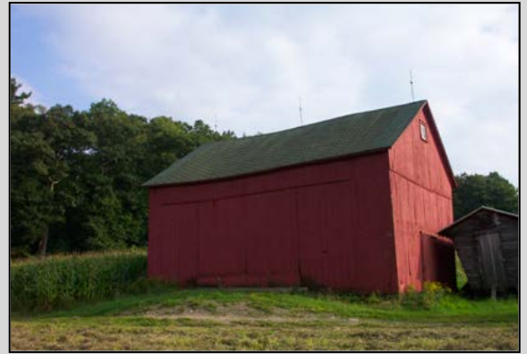
English barn, Ransom Township, Lackawanna County, c. 1860-1890. Site 069-RA-001.
