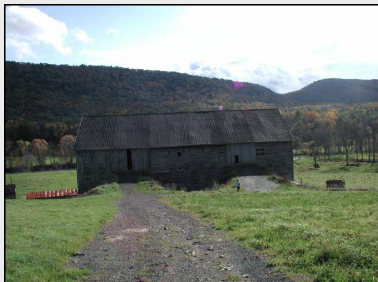
Hodge Barn, Centre County, struts under forebay.
