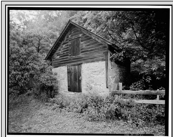
Ice house, Walter-Kautz Farm, Smithfield Township, Monroe County, c. 1880. Photographed by George Eisenman in 1968. Historic American Buildings Survey, digital ID http://hdl.loc.gov/loc.pnp/hhh.pa0615 .
