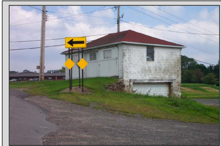
Root storage building, Dallas Township, Luzerne County, c. 1920-40. Site 079-DA-001.
