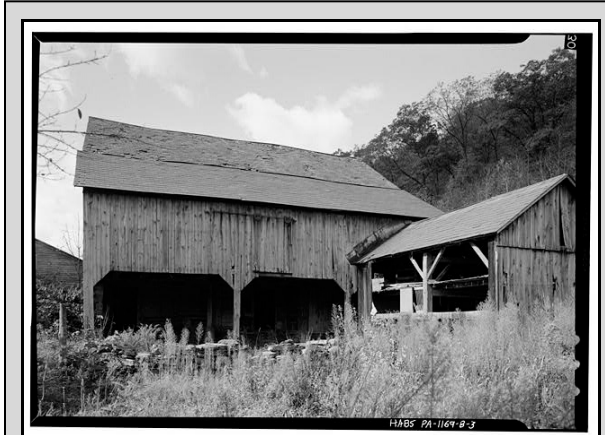
Walter-Kautz Farm, Barn, Smithfield Township, Monroe County, c. 1877. Photographed by Jack E. Boucher in 1969. Historic American Buildings Survey, digital ID http://hdl.loc.gov/loc.pnp/hhh.pa0613 . The floor plan below shows how a Pennsylvania forebay barn was converted to this barn.
