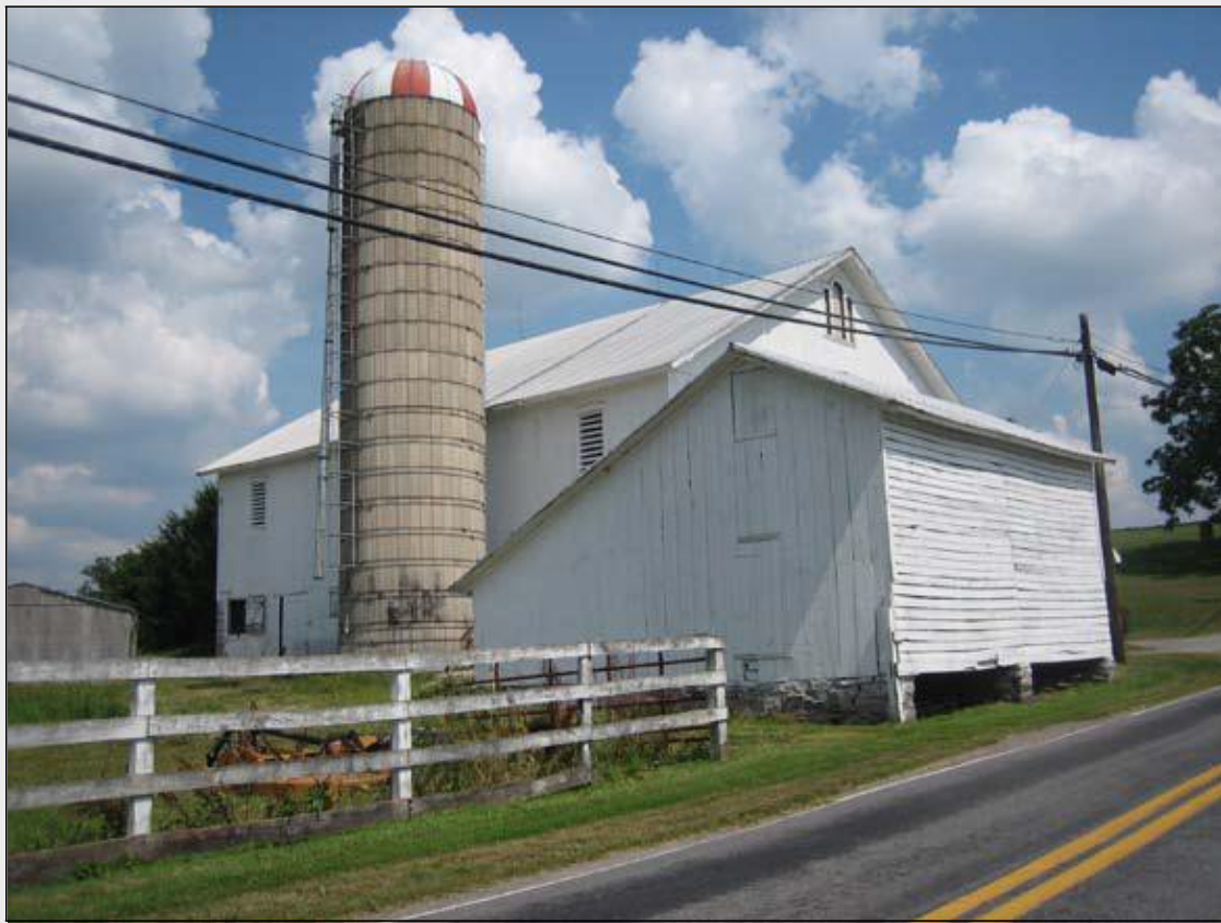
Corrugated concrete stave silo, Jackson Township, Dauphin County, c. 1945-65. Site 043-JA-007.
