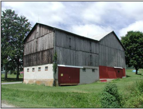
Three-Gable Barn with lower level altered for dairy, Greenwood Township, Columbia County, original barn c. 1900, alterations c. 1950. Site 037-GR-002.
