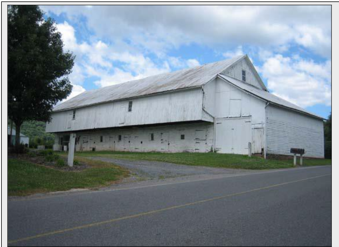
Pennsylvania barn with shed roof machine shed/corncrib addition, Reed Township, Dauphin County, c. 1860 and c. 1900. Site 043-RE-001.
