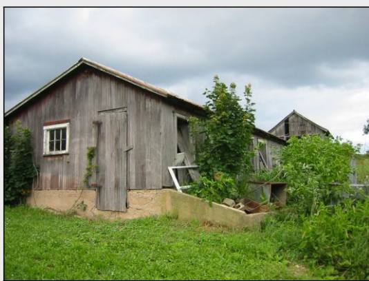
Hog house,, Locust Township, Columbia County, c. 1930-45. Site 037-LO- 004.
