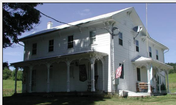
One room deep four-over-four house, Greenwood Township, Columbia County, c. 1850. Site 037-GR-005.
