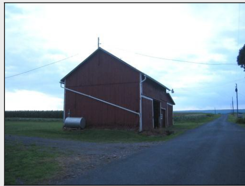
Machine shed, Locust Township, Columbia County, c. 1930. Site 037-LO-007.
