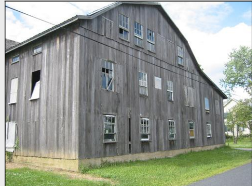
Three-Gable Barn adapted for poultry, Locust Township, Columbia County, original barn c. 1920, adaptations c. 1950. Site 037-LO-003.
