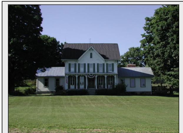
Five bay house updated with center gable, French doors, 2/2 windows, and bracketed porch and cornice, Greenwood Township, Columbia County, c. 1867. Site 037- GR-006.
