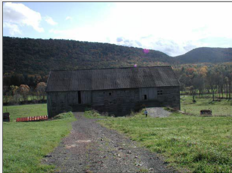
Hodge Barn, Centre County, struts under forebay
