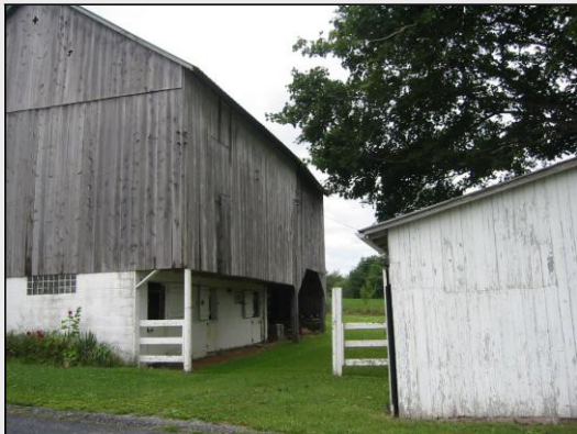
Pennsylvania forebay barn with machinery bay, Locust Township, Columbia County, late 19 th century. Site 037-LO-001.
