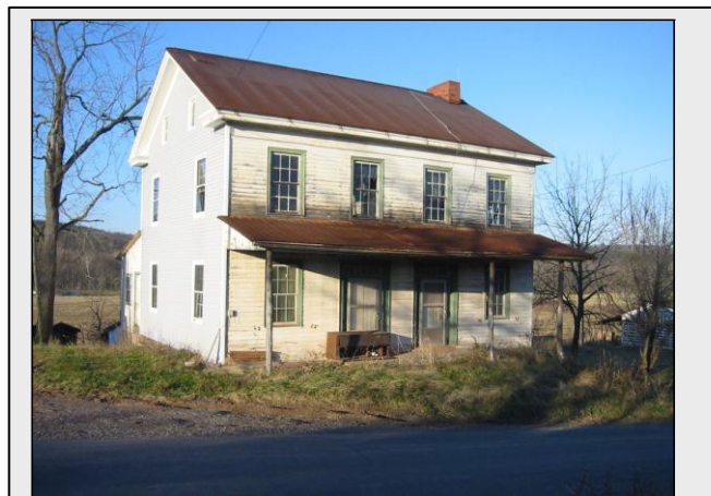
Four-over-four house with two doors, Middleburg Township, Snyder County, c. 1840-60. Site 109-MI-001.
