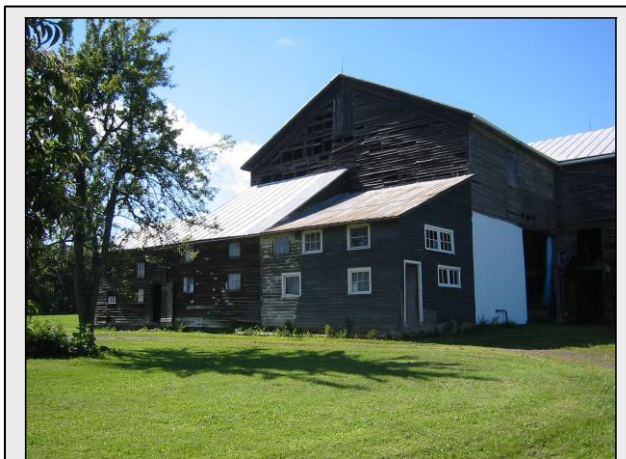
Three-Gable Barn with shed roof poultry additions, Greenwood Township, Columbia County, Site #005.
