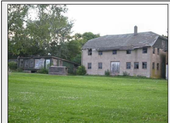
Poultry houses, Locust Township, Columbia County, mid 20 th century. Site 037-LO-006.
