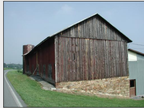
Log and frame forebay barn, Lower Mahanoy Township, Northumberland County, 1845. Site 097-LM-005.
