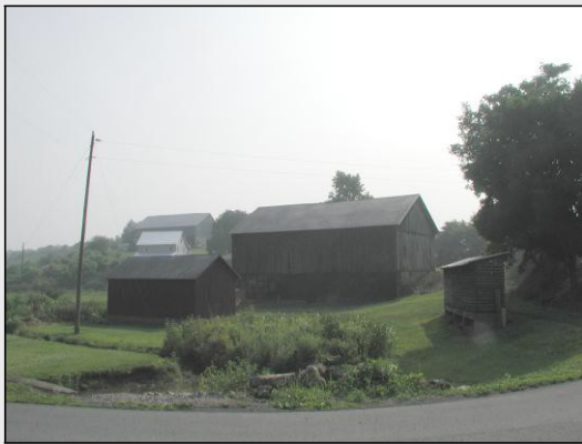
Pennsylvania Barn, Lower Mahanoy Township, Northumberland County, mid 19 th century. Site 097-LM-006.
