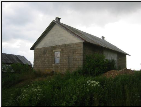
Molded concrete brick machine shed with ground level root cellar, Locust Township, Columbia County, c. 1930. Site 037-LO-004.
