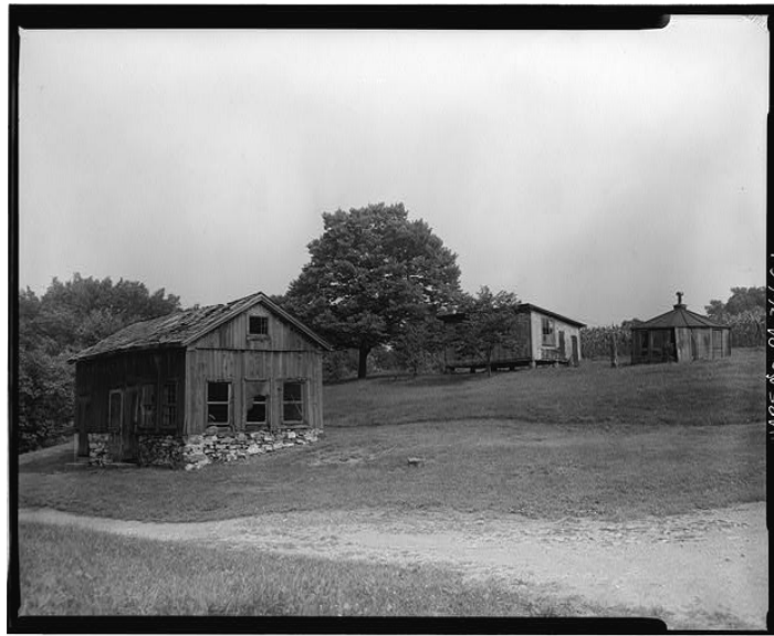
“Chicken and brooder houses,” Stamm Farm, Penn Township, Berks County. According to the HABS documentation, the house in the foreground is the oldest, but no date is given. The shed roof building in the background was probably built in the mid-twentieth century; it stands on concrete piers that were made by pouring wet concrete into barrels. The brooder house at right is a metal building, probably prefabricated. These “peepy” houses were popular in the early twentieth century. Digital ID http://hdl.loc.gov/loc.pnp/hhh.pa0163
