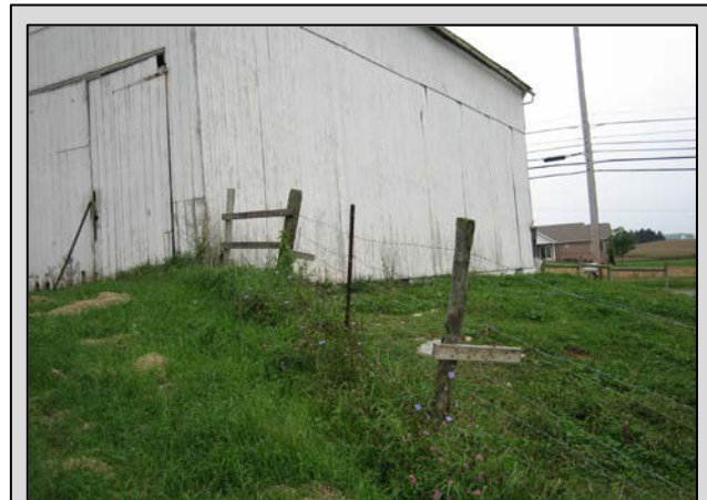
Barbed wire fencing, Jackson Township, Lebanon County, date unknown. Site 075-JA-008.
