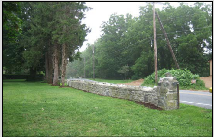
Fence and tree windbreak, Mill Creek Township, Lebanon County. The fence has an incised date of 1851, but it is cut into a later concrete reinforcement. Site 075-MC-001.
