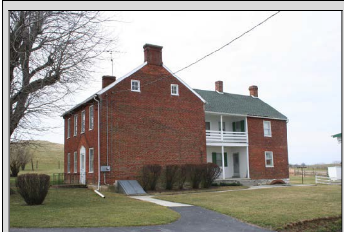
Brick-cased log house, Washington Township, Franklin County. The main section was built around 1820 and cased with brick around 1850; the ell was added later in the nineteenth century. Site 055-WA-003.
