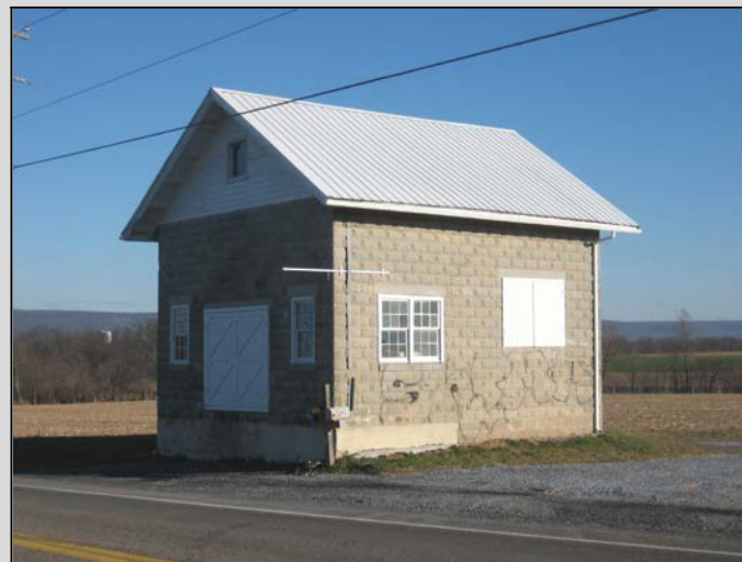
Milk station, Tulpehocken Township, Berks County, c. 1940. This building is located along Route 501 at the end of a long farm lane.
