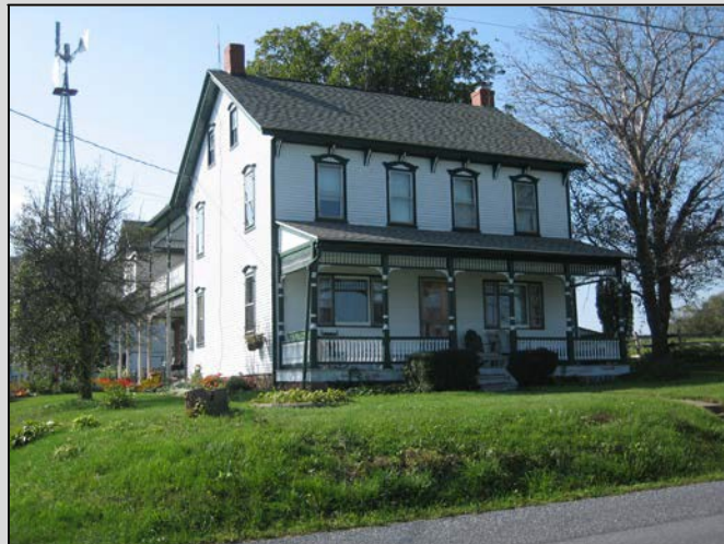
Four over four house with Victorian trim, Bethel Township, Lebanon County, c. 1875-90. Site 075-BE-001.
