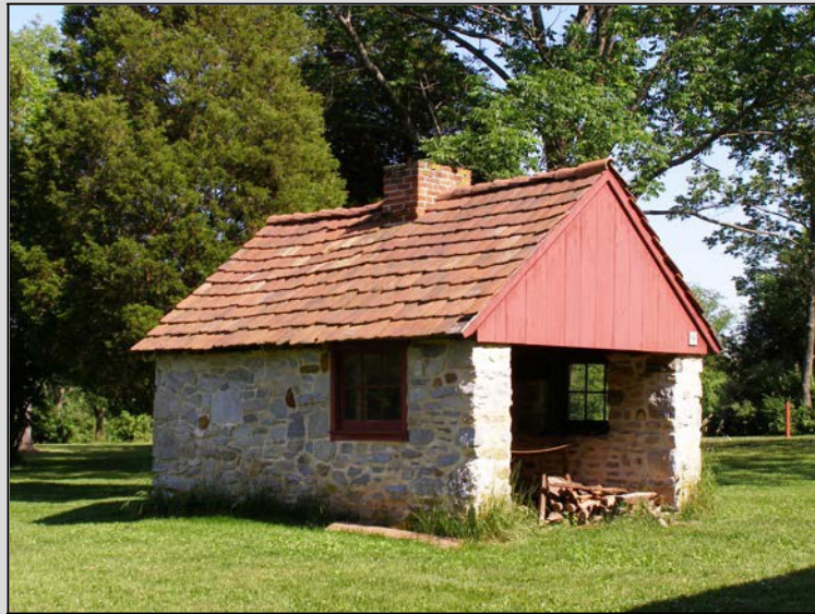
Bakehouse, Bertolet-Herbein homestead, Berks County, reconstructed, date uncertain. The bake oven was situated in the rear, but a “squirrel” tail ran the smoke back into a chimney on the roof ridge. A sheltered area protected workers and products.
