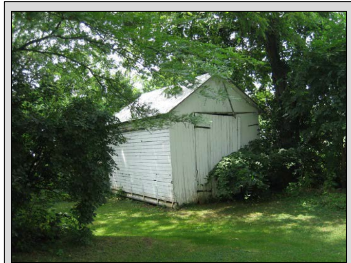
Corn crib, Heidelberg Township, Lebanon County, c. 1940. A late example of canted sides. Site 075-HE-001.
