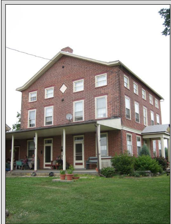
House with formal Georgian front and informal gable end entry, South Annville Township, Lebanon County, built by Commodore Perry Steinmetz in 1852. West gable end. This was the kitchen side and faced the working part of the farm. Site 075-SA-006.
