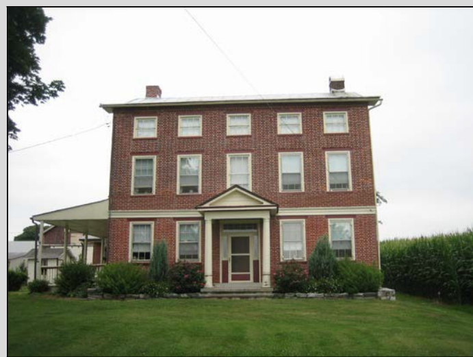
House with formal Georgian front and informal gable end entry, South Annville Township, Lebanon County, built by Commodore Perry Steinmetz in 1852. South eaves side. This was the “public” front. Site 075-SA-006.
