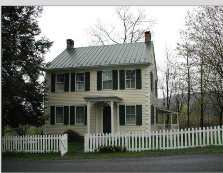
Four over four house, Oley Township, Berks County, c. 1870. The corner quoins, window trim, 2/2 sash, and porch ornament give the form an updated look.
