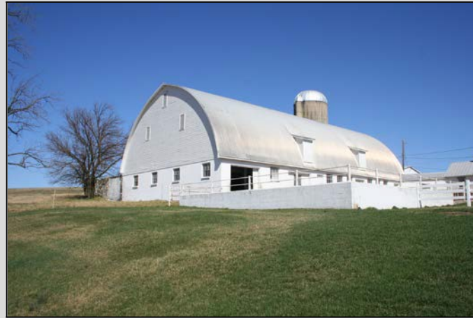
Stable barn, Straban Township, Franklin County, mid- to late twentieth century barn built on earlier stone foundation. This barn retains the barnyard wall characteristic of the Pennsylvania forebay barn, only it is built of concrete block and metal pipe. Site 055-ST-003.
