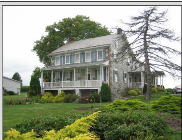
Five-bay house with center door and walk-in lower level, South Annville Township, Lebanon County, 1855. The lower level has a spring house and kitchen, and is connected to the first floor by a dumbwaiter. Site 055-AN-005.
