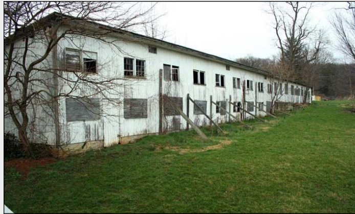
Chicken house at Landis Valley Museum, Lancaster County, early twentieth century.
