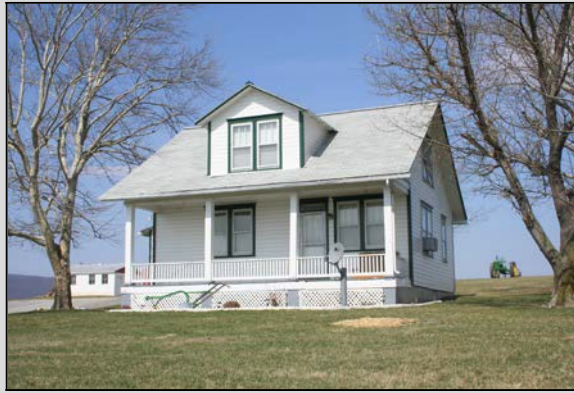
Bungalow, Lurgan Township, Franklin County, c. 1925-1940. Site 055-LU-001.
