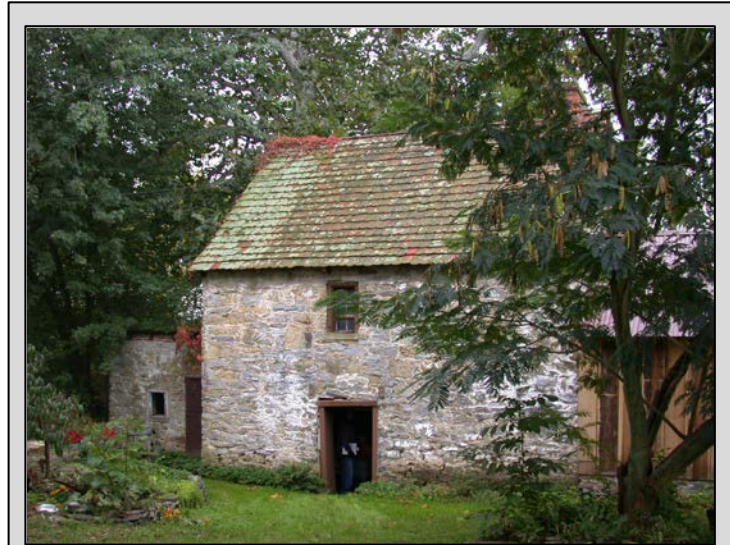
Abraham Bertolet ancillary house, Oley Township, Berks County, c. 1740. This building had a first story kitchen.
