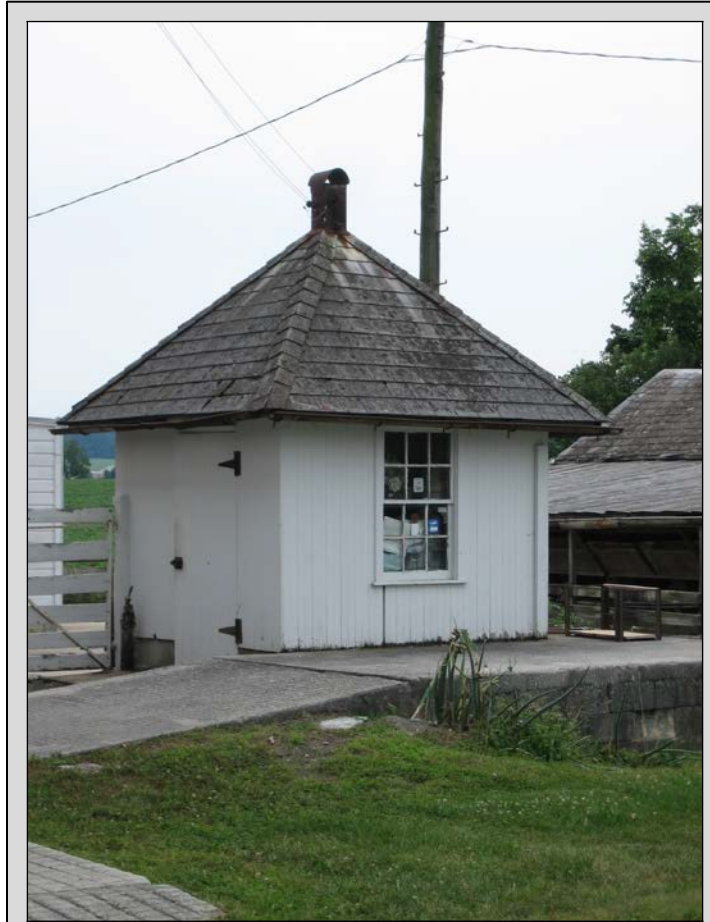
Pump house, South Annville Township, Lebanon County, c. 1930-40. Site 075-SA-004. This pump house function was given by someone familiar with the site. It sits on a concrete platform in the barn yard, about twenty-five feet from the barn forebay. This site also has a milk house, sited at the barn's gable end directly on the farm lane.
