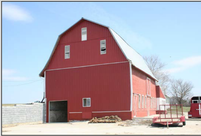
Stable barn, Lurgan Township, Franklin County, c. 1950. Site 055-LU-001.
