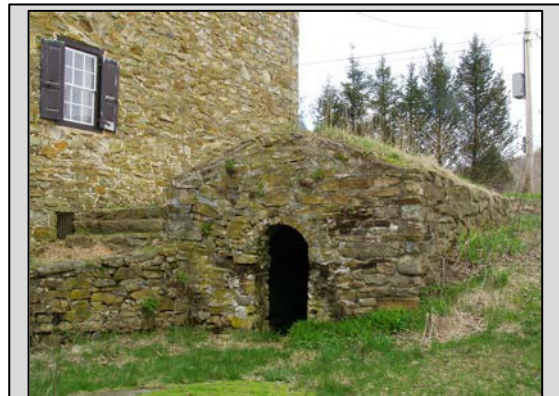
Root cellar, Keim homestead, Oley Township, Berks County, early nineteenth century.
