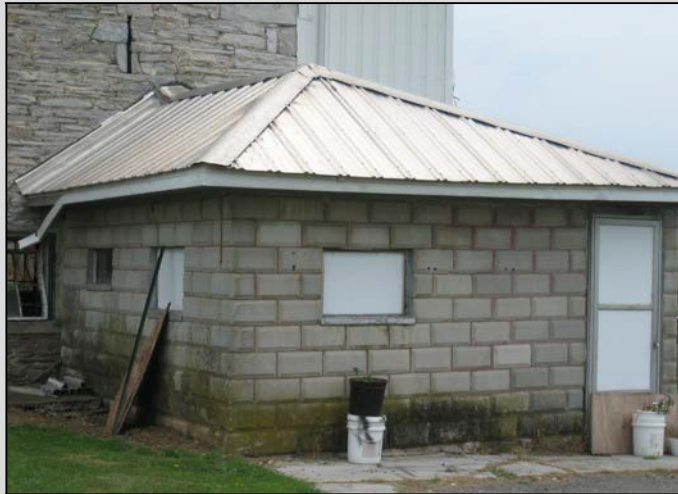
Beveled block milk house, North Cornwall Township, Lebanon County, c. 1930-1940. Site 075-NC-002.
