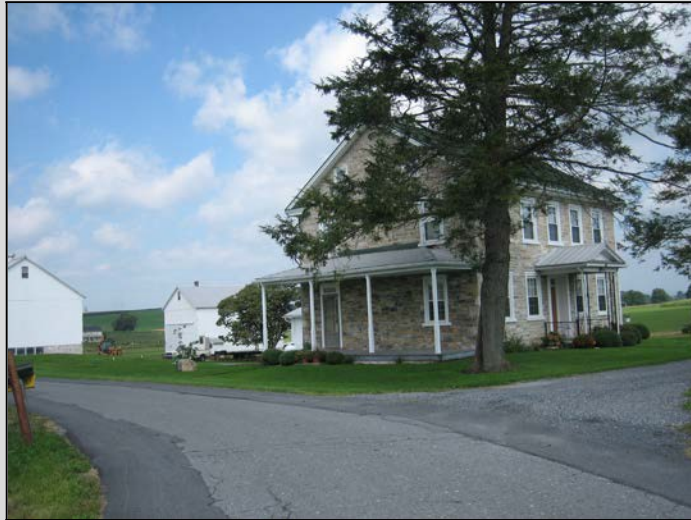
House with formal Georgian front and informal gable end entry. The porch and tree obscure it a little, but the gable-end entrance leads to a kitchen and the front is symmetrical and more formally trimmed. Mill Creek Township, Lebanon County, c. 1855. Site 075-MC-011.
