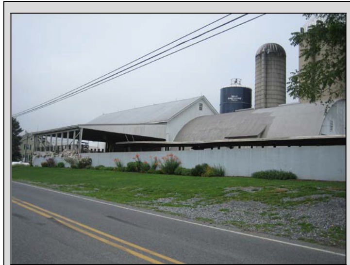
Pennsylvania barn with shed-roof loafing area addition and rainbow-roof stable barn addition, Mill Creek Township, Lebanon County, nineteenth century original with mid-twentieth century modifications. Site 075-MC-006.
