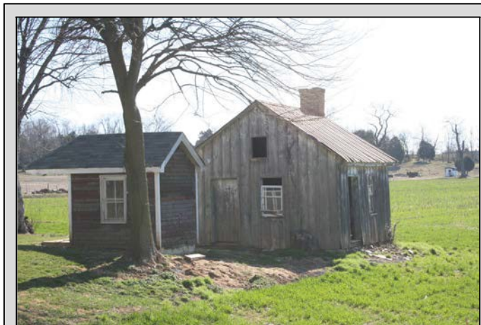
Pump house (foreground) and summer kitchen, Antrim Township, Franklin County, c. 1910-40. Note the small size, extended roof for added protection from the weather, and the location next to a summer kitchen.
