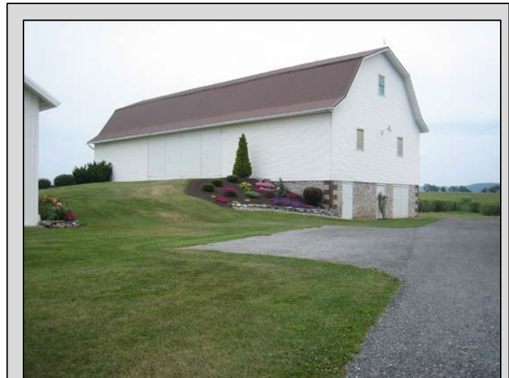
Pennsylvania barn transformed into a gambrel-roof stable barn, South Annville Township, Lebanon County. Original construction probably c. 1850; modified in the mid-twentieth century. Site 075-SA-002.
