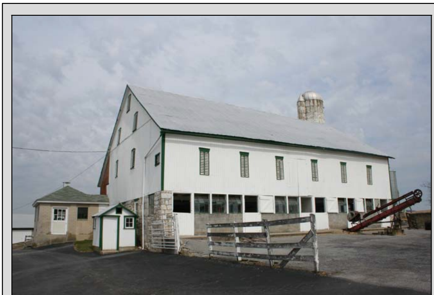
Pennsylvania forebay barn adapted for dairy, Washington Township, Franklin County. Original construction late nineteenth century, adapted early twentieth century. Note the canted metal framed windows combined with concrete block wall and traditional Dutch doors. Site 055-WA-003.
