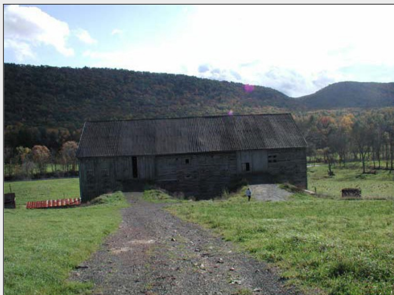
Hodge Barn, Centre County, struts under forebay
