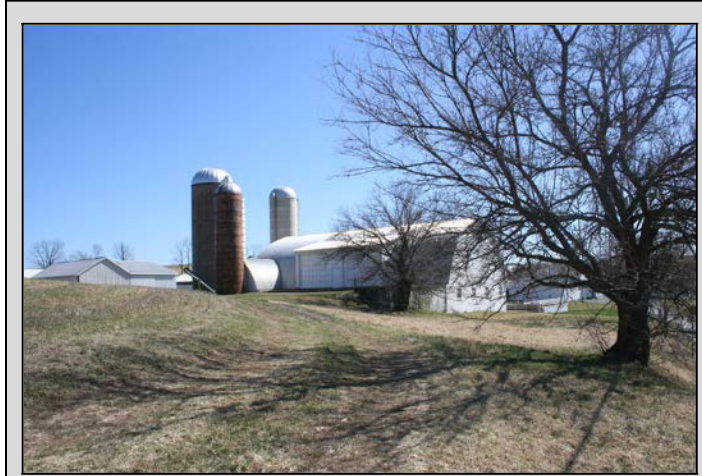
Metal silo, concrete stave silo, and poured concrete silo, Straban Township, Franklin County, c. 1940, 1950, 1970 respectively. Site 055-ST-003.
