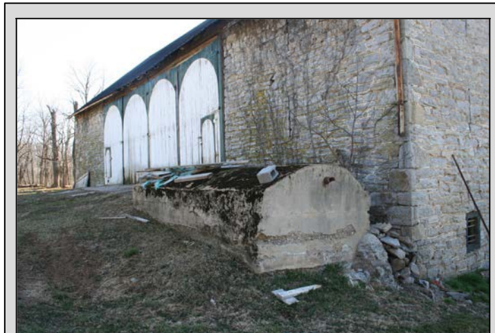
Cistern, Antrim Township, Franklin County, early twentieth century. Site 055-AN-005.
