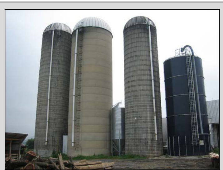
Three types of silo: from left to right, concrete stave, poured concrete, concrete stave, and Harvester. The concrete stave silos are probably mid-twentieth century and the others more recent. Mill Creek Township, Lebanon County. Site 075-MC-006.
