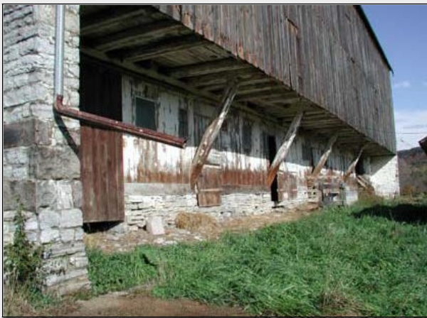
Hodge Barn, Centre County, struts under forebay
