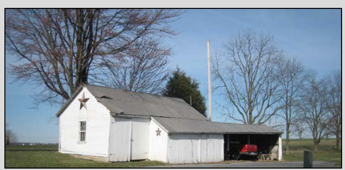
Machine shed, Antrim Township, Franklin County, c. 1925-45. Site 055-AN-011.
