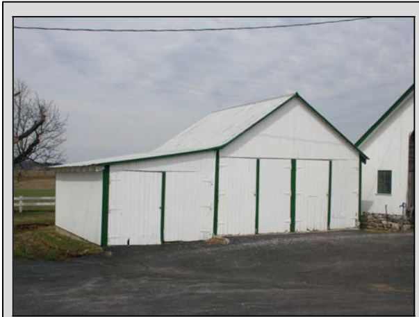
Garage, Washington Township, Franklin County, c. 1920-35. This building may have originally been a carriage house. Site 055-WA-003.
