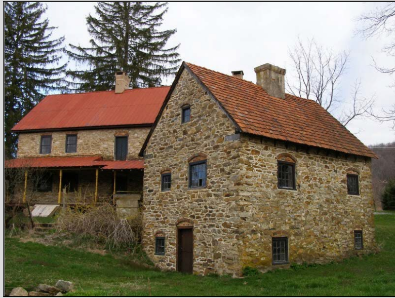
Keim Homestead ancillary building, Oley Township, Berks County, c. 1760. This banked structure had a spring in the basement and accommodated a wood-turner shop on the upper level.
