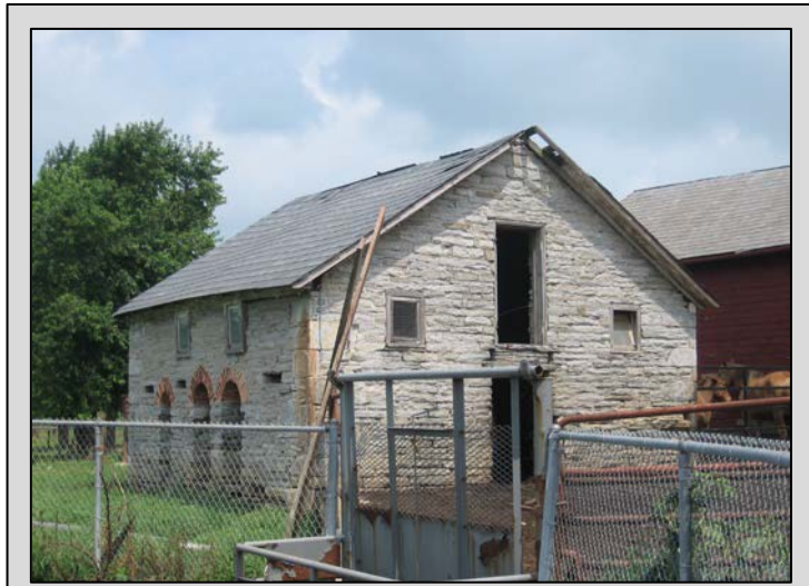
Pigsty, Heidelberg Township, Lebanon County, c. 1865-75. A rare stone example with decorative brick arches over the doors. Site 075-HE-006.
