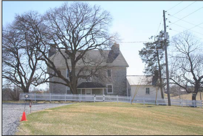
Farmhouse with shade trees and picket fence, Straban Township, Franklin County. The fence is new, but the trees are mature. Site 055-ST-003.
