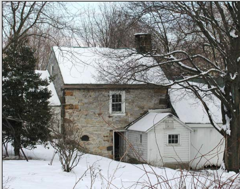
Spring house, Cumberland County, late eighteenth or early nineteenth century. This combination building has a spring in the basement and a fireplace on the upper level.
