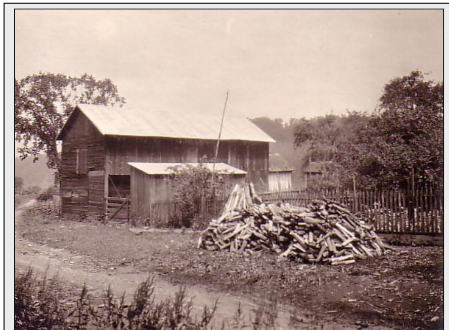
This Juniata County building, from an undated photo, may be a hog house. The evidence: scale, linear arrangement with respect to yard, windowless lower level, fenced in area. Juniata County Gen Web site.
