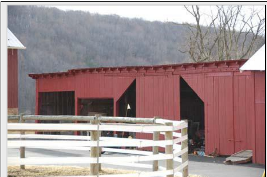
Wagon Shed, Bedford Township, Bedford County, c. 1910. Site 009-BED-002.
