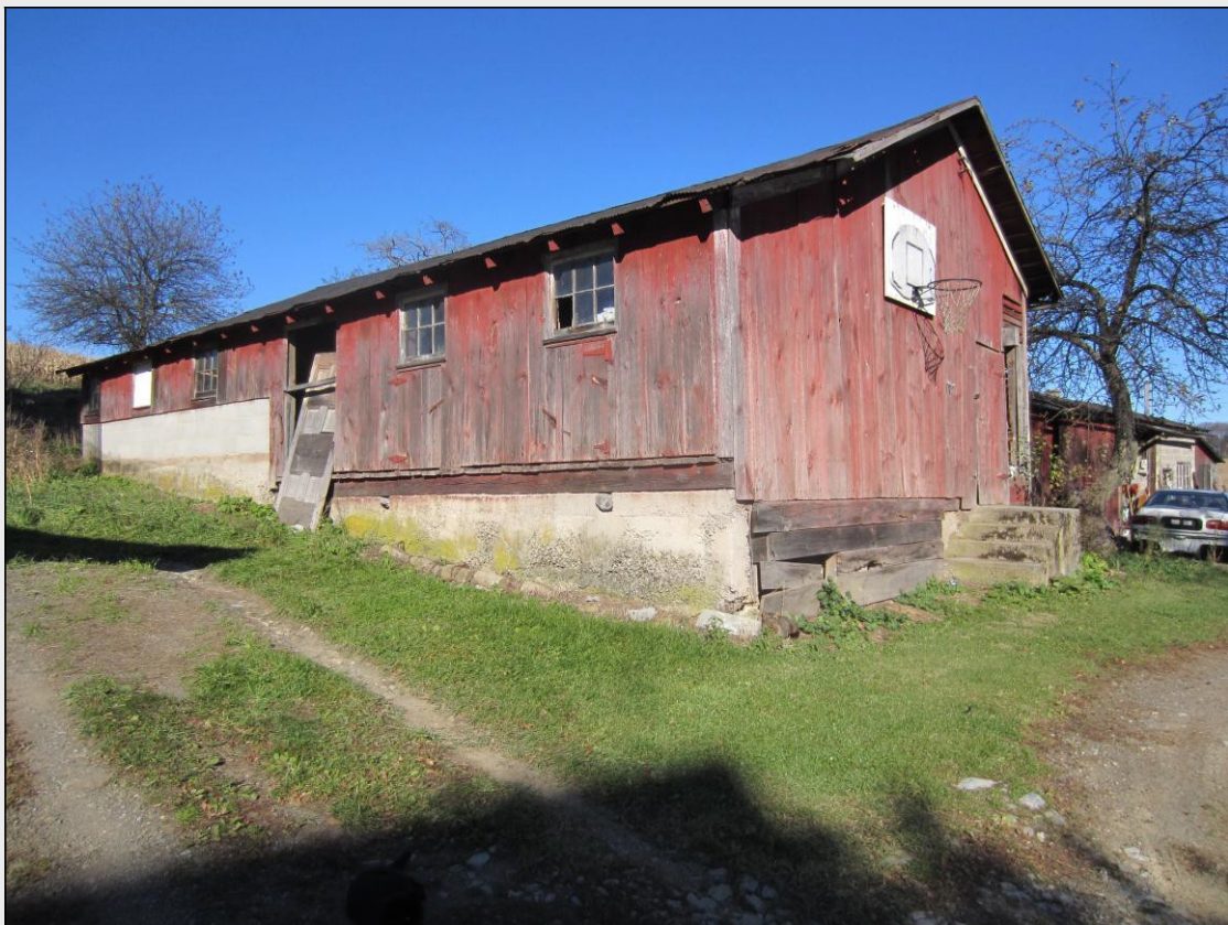
Hog house, Potter Township, Centre County, date unknown. The building has the trademark features of asymmetrical gable roof and gable-end human entryway leading to feed aisle.
