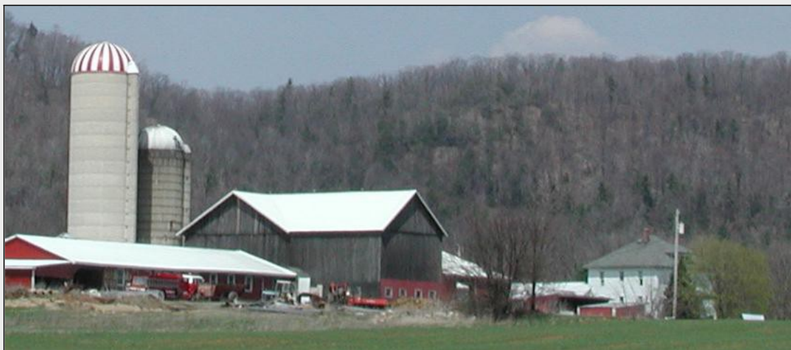
Farmstead, Potter Township, Centre County. This picture illustrates some of the key changes of the 20th century: poured concrete and concrete stave silos; three gable barn altered for dairy (note the windows cut into the lower level); pole barn (post war); foursquare house.
