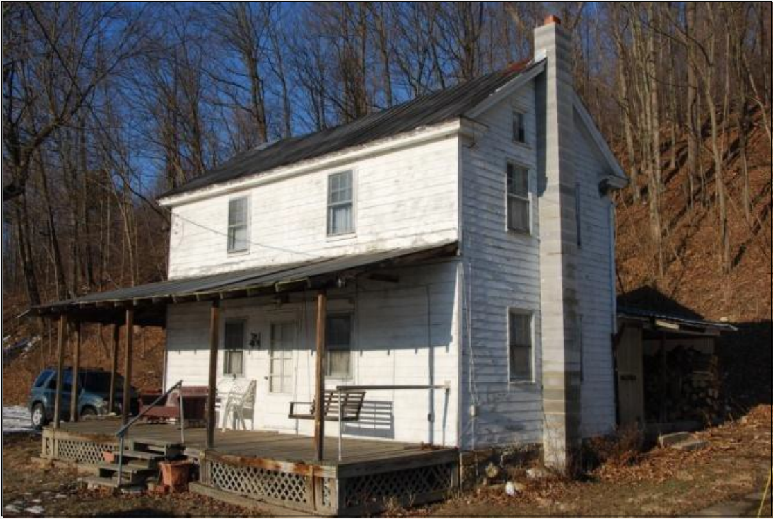
House, East Saint Clair Township, Bedford County, c. 1840-1860. Site 009-ESC-003.
