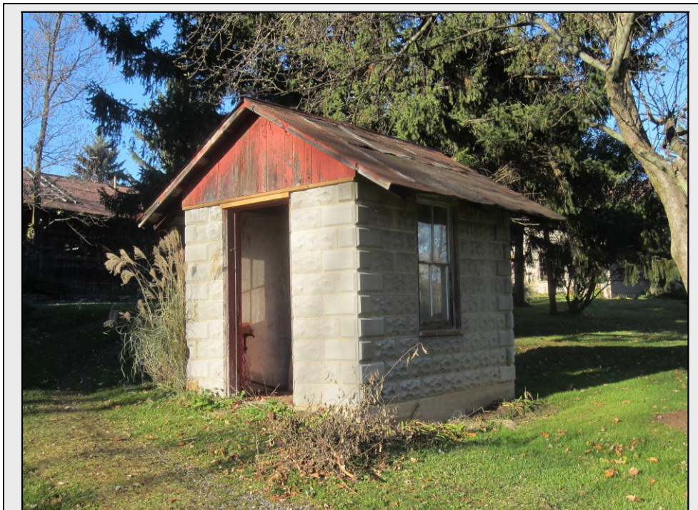
Rockface concrete block milkhouse, Potter Township, Centre County, c. 1935. Photo-only site, no site number.
