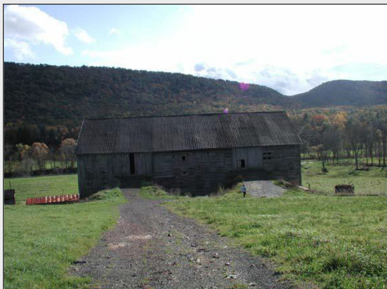
Hodge Barn, Centre County, struts under forebay
