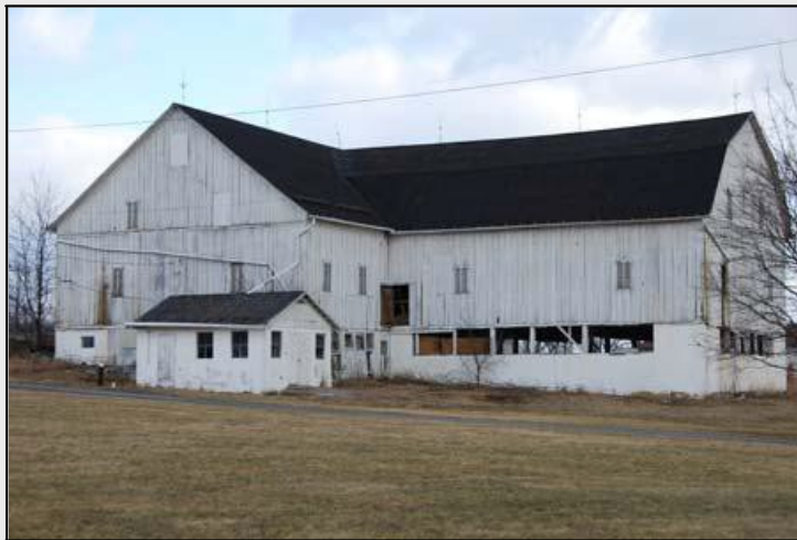
Extended forebay or basement Barn with free-stall gambrel roof extension, Colerain Township, Bedford County, late 19th-early 20th century.
