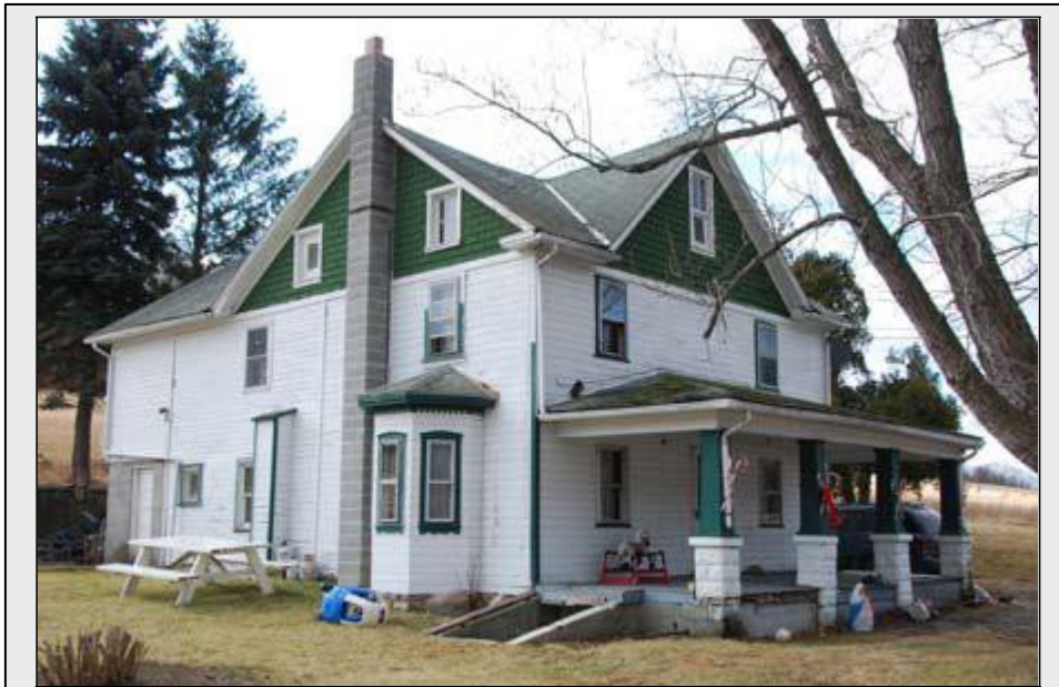
Center-gable house, Bedford Township, Bedford County, c. 1879-1890. Site 009-BED-001.
