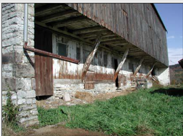
Hodge Barn, Centre County, struts under forebay
