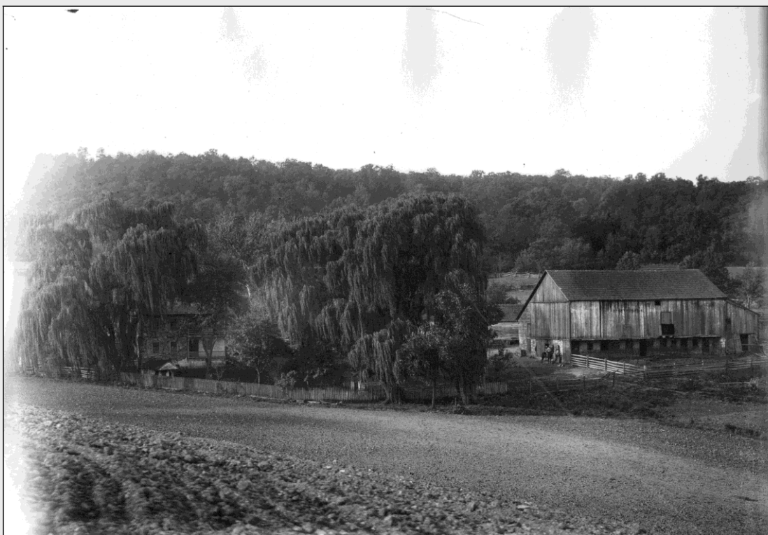
Farmstead, probably in Mifflin County, late 19th-early 20th century. Note the ornamental willow trees, picket fence around the house, board fence around the barn yard, and Pennsylvania forebay barn. Francis Cooper Collection, Pennsylvania State Archives MG 464 Box 1, photo #FC164.
