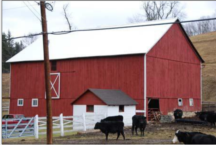
Basement or extended-forebay barn, Napier Township, Bedford County, 19th century. Site 009-NAP-001.
