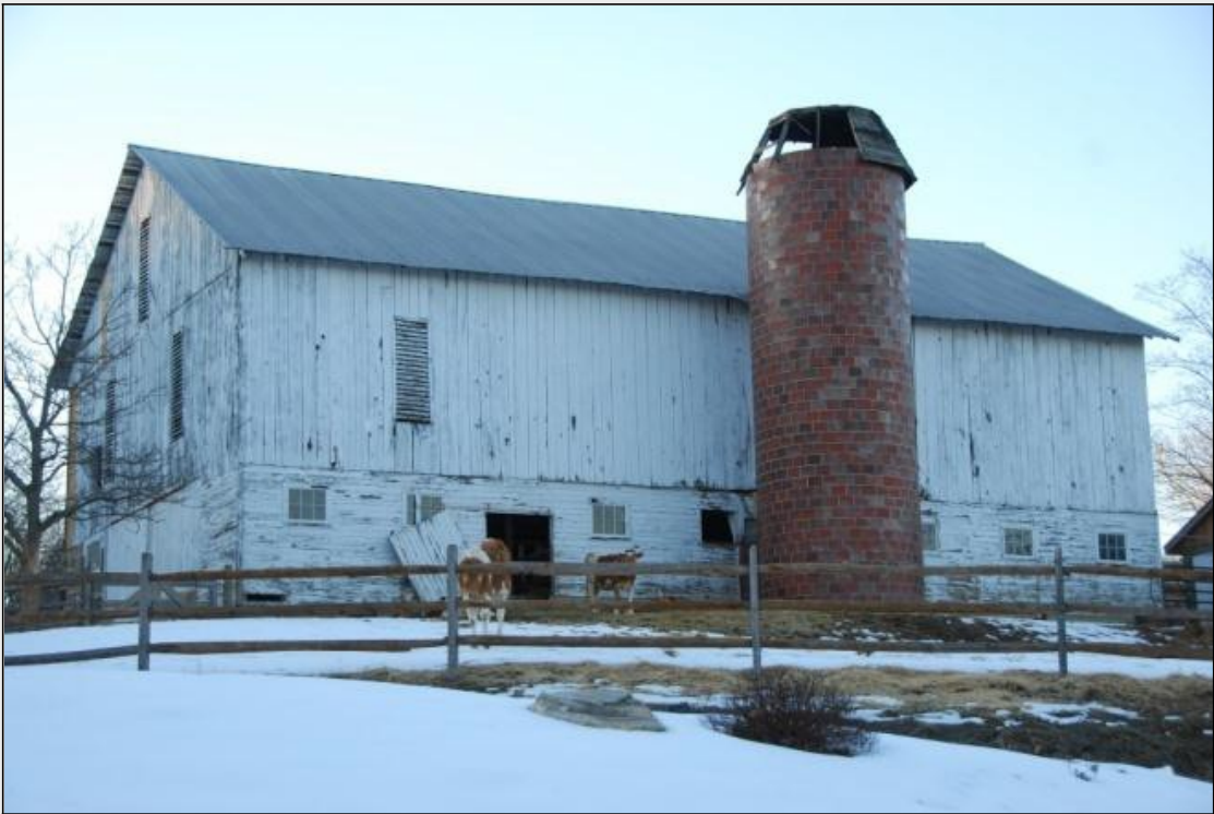
Basement or extended forebay barn, East Saint Clair Township, Bedford County, 19th century. Site 009-ESC-007.
